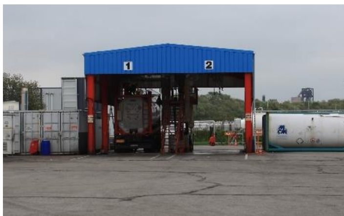
Station de lavage
